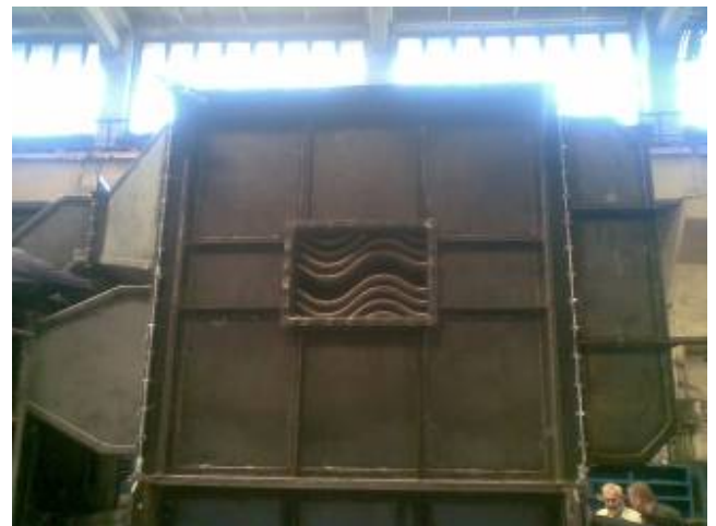
Fig.5. View of the air pre-heater's pipes beam.
